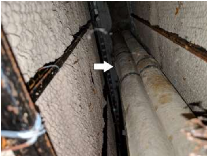
ACM- Pipe insulation (T.S.I)
