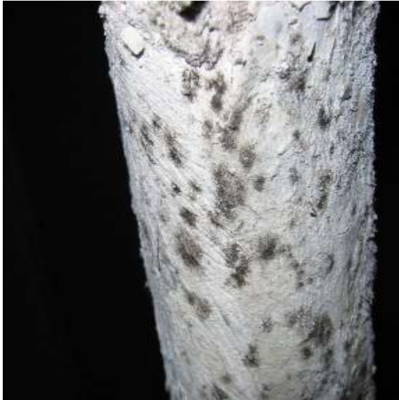
ACM- Pipe insulation (T.S.I)
