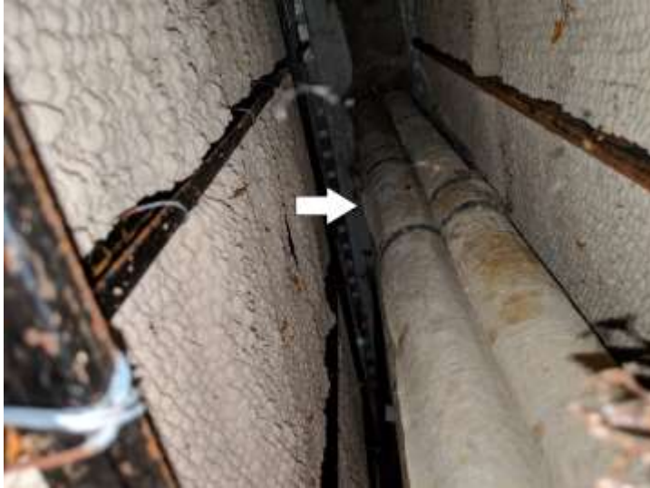
ACM Pipe insulation
